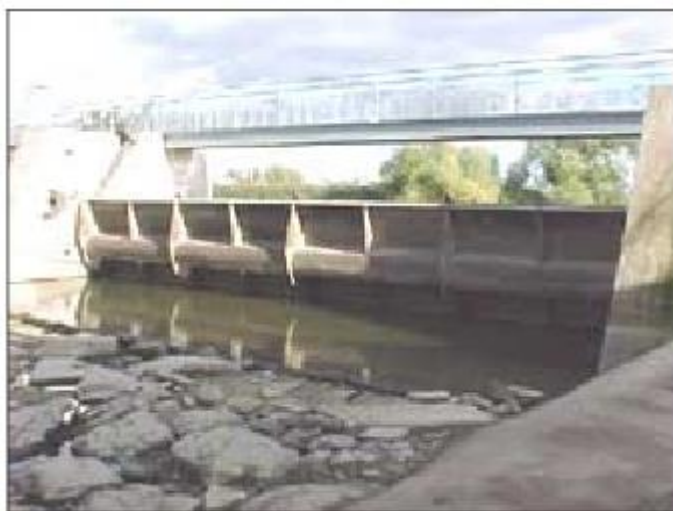
Clapet type tube de torsion
